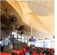
tremely economical, climatic regulation. In summer, large air masses are moved downwards during normal operation. By controlling the speed of rotation, warm pent-up air is gently guided from the ceiling to the ground in winter (destratification).
